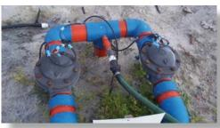
Figure 2. Injection point with hose coming from the nurse tank in Figure 1.
