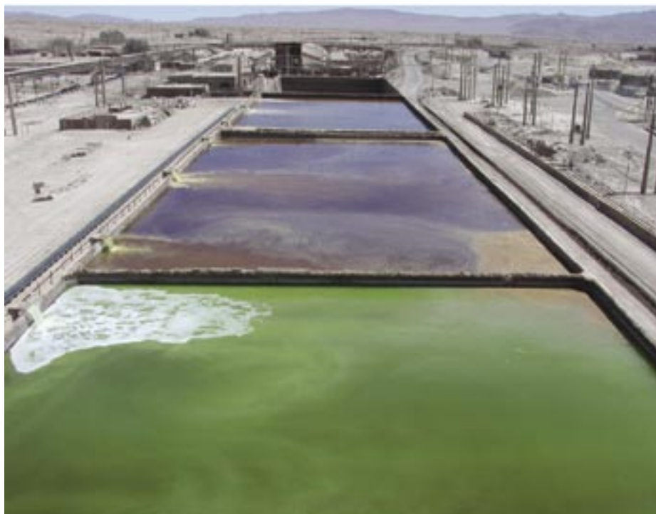
Figure 22: Closed counter current extraction vats
