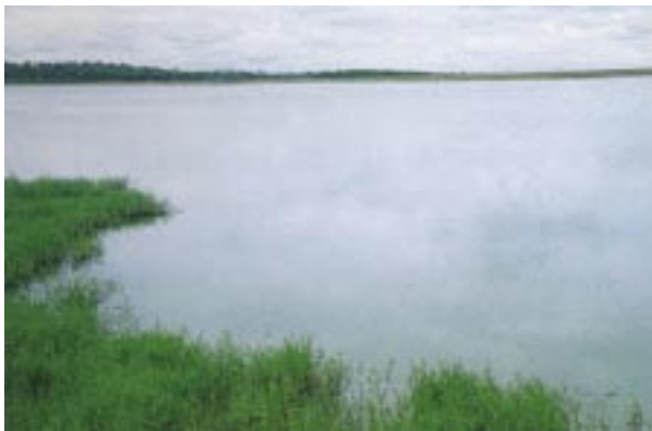
Tailingsdam, wall in distance – Copebras S.A. Brazil
